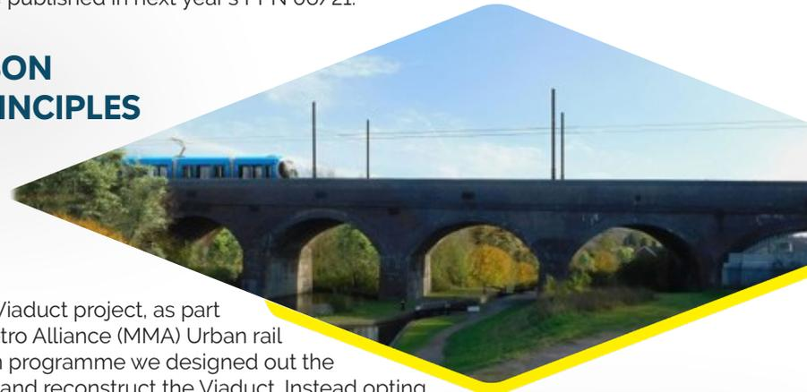
On our Parkhead Viaduct project, as part of the Midland Metro Alliance (MMA) Urban rail network extension programme we designed out the need to demolish and reconstruct the Viaduct. Instead opting for a refurbishment design which saved over 1500 tCO2e through the reduction in materials, such as concrete and steel.
